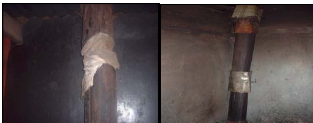
Figure 3 Methods of sealing chimneys
